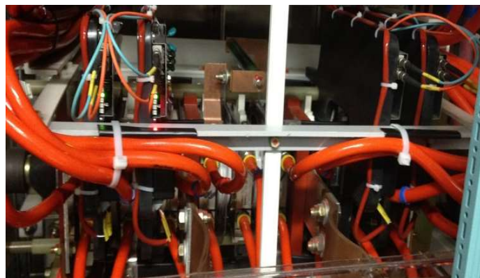
New hoses after replacement
